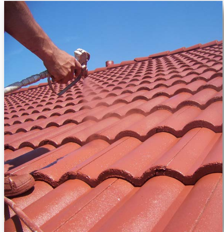
IR Heat-Reflective PVDF Coating applied to tile roof surface
